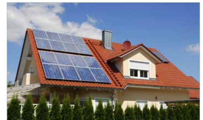
Solar heating systems (collectors)
