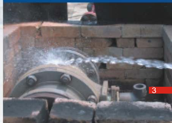
Valve after Test
